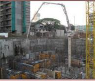
The Orchid Crown project site at Mumbai has achieved the pumping of M-80 grade concrete by pumping it with a BP 2800 concrete pump through 600m concrete pipeline. This is the longest length of pipeline and highest grade of concrete pumped so far among Buildings & Factories sites of L&T. The site has pumped 2500cu.m of M-80 grade concrete so far. Apart from this the site has completed 30,000cu.m of M-60 grade concreting in the last eight months.
