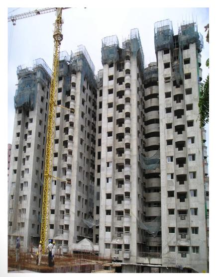
Concrete of SCC type with M 30 Grade for Residential Towers at Hyderabad. The site was adjudged Outstanding Concrete Structure by ICI, Hyderabad
